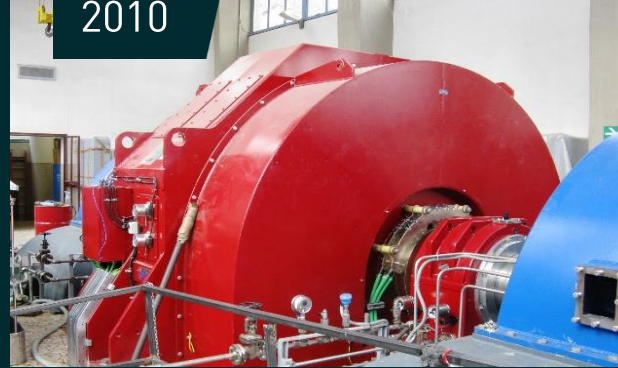
HPP Albano, Italy 19000 kVA, 6300 V, 500 rpm Double Pelton Turbine
