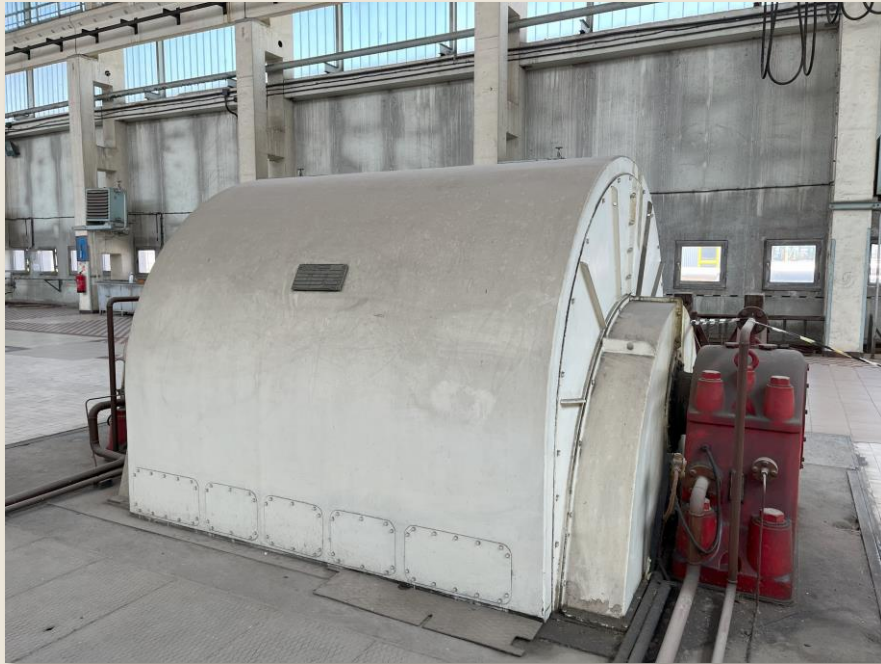
Kazincbarcika TPP, Hungary ON 1300x1250/6 11500 kVAr 6300 V 1055 A 50 Hz 1000 rpm
