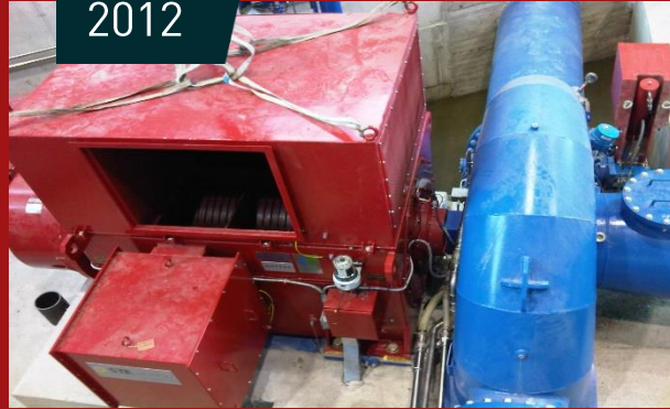
HPP Temu, Italy 2x 2 900 kVA, 6.3 kV, 750 rpm, IM B3, IC 21 Francis Turbine
