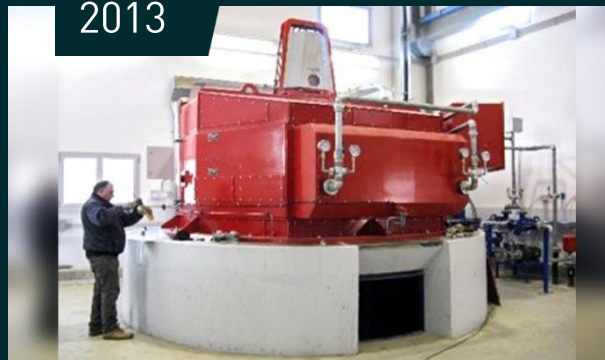
HPP CREMA 1200 kVA, 40P, 150 rpm, V1 – Onv 2660x275/40 Kaplan Turbine
