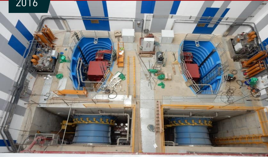
HPP South Maris Canal, Philippines 2 x 5000 kVA, 10P - 720 rpm - Pit Kaplan Turbines
