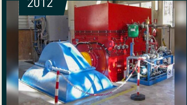
HPP COGNO, Italy 3x 2400 kVA, 6P - SRGb 636Ks6 Pelton Turbine
