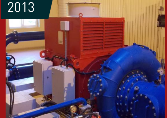
Compact container unit 610 kVA, 0.4 kV, 1000 rpm, IM B3, IC 01 Francis Turbine
