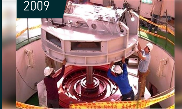
HPP Zho Tuwei, Taiwan 4000 kVA, 30 pole, V1 ONv2600L30 Kaplan Turbine
