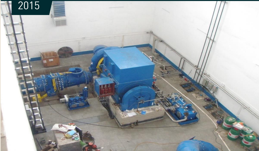
HPP Song Quang, Vietnam 2x 7 781 kVA, 6.3 kV, 750 rpm, IM B3, IC 81W7 Francis Turbine
