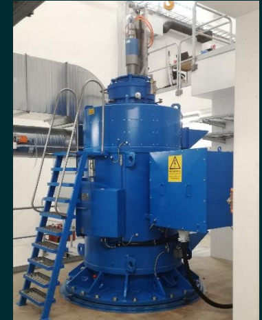
HPP Tanfallet, Sweden 2.4 MVA, 750 rpm Kaplan Turbine
